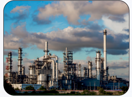
Acid & Chemical Plant
